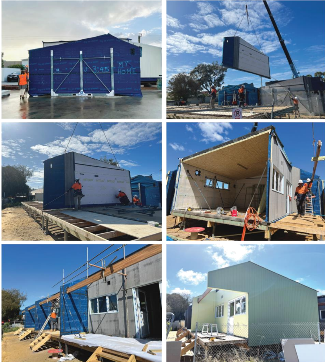
Sequence of construction at the "My Home" North Fremantle site. Completion: March 2023
