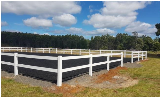
L. Example of post and 2-rail fencing
